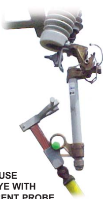
STEP 2 CAPTURE FUSE TUBE WITH FUSE CLAW WITH FORWARD MOTION
